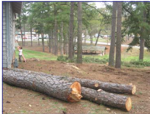
Trees being removed from beside the Hut.
